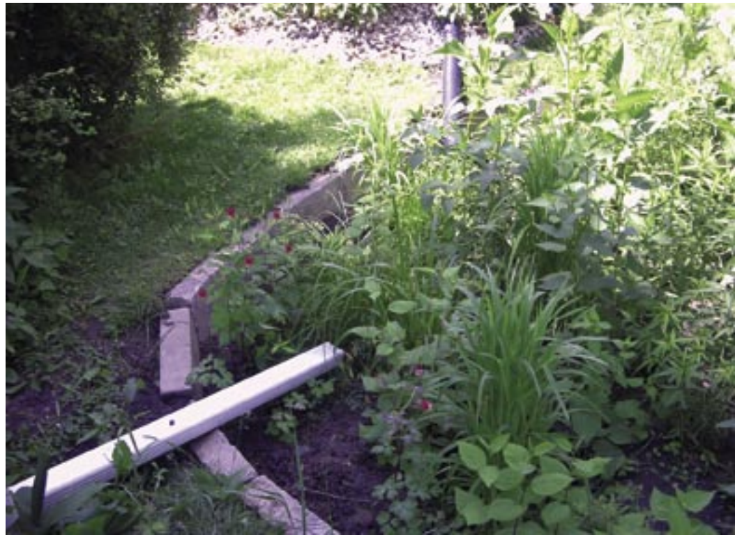
Figure 9. Rain garden. Photo: S. Jones, Dane Co. Land and Water Resources Dept.
